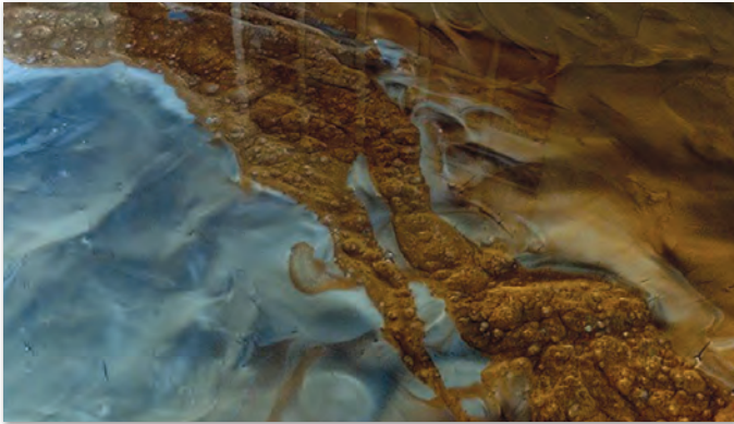
Epoxy Metallic Floor
