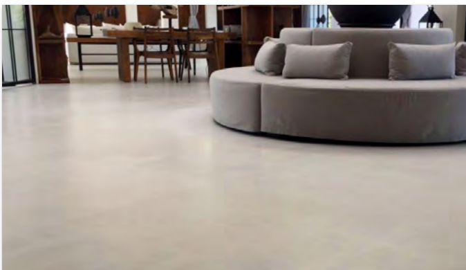
Interior Concrete Overlay
